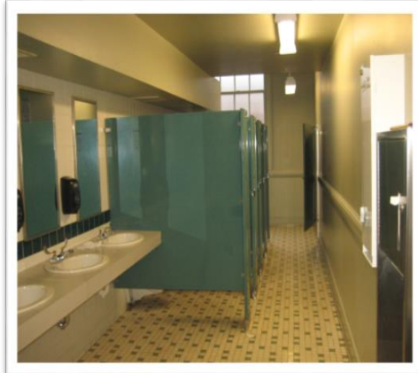
Old Cabell – Bathroom before
