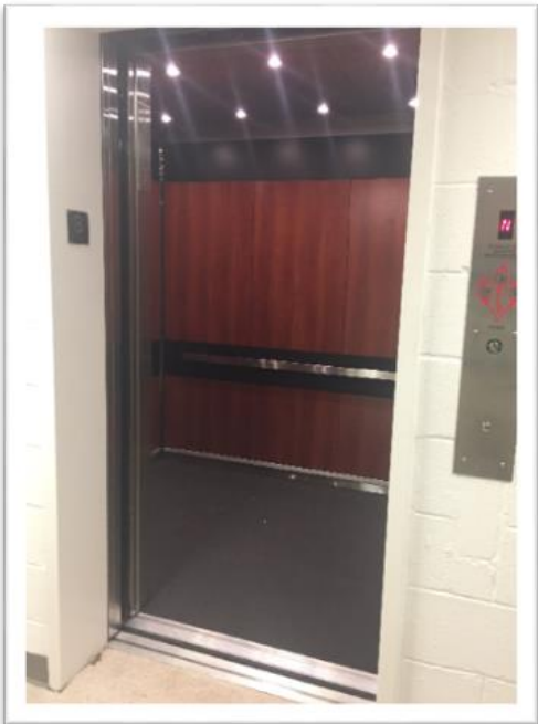
Withers Brown – Elevator Modernization Completed
