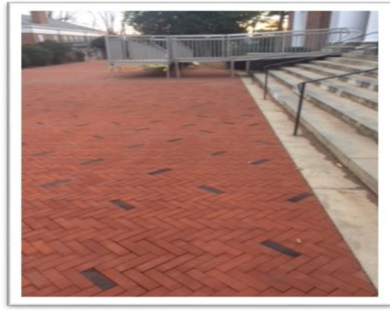
Clark Hall Plaza - After
