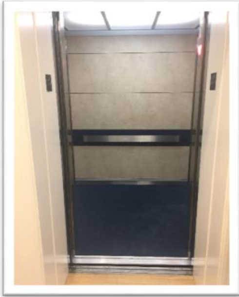
Peabody Hall – Elevator modernization after
