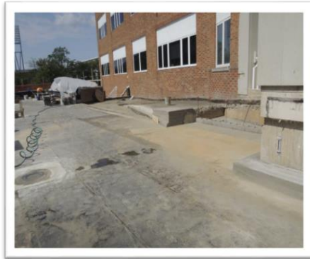
Chemistry Plaza – Removal of old water proofing
