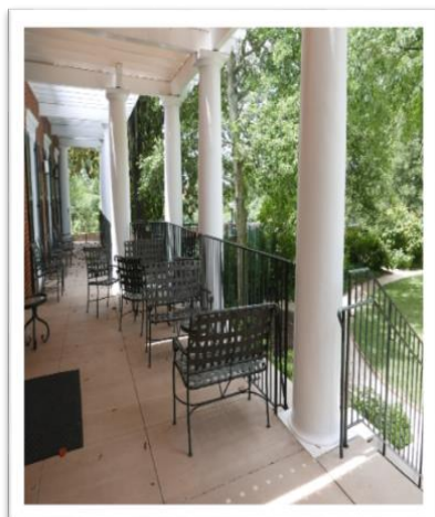
Pav. VII Porch - Before
