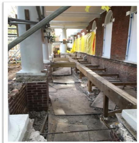
Pav. VII - In progress (removed)
