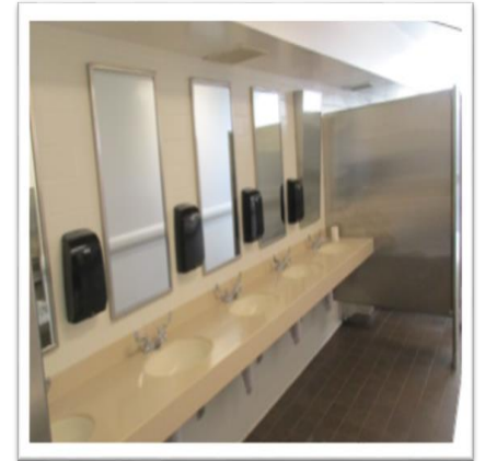
Old Cabell – Bathroom after
