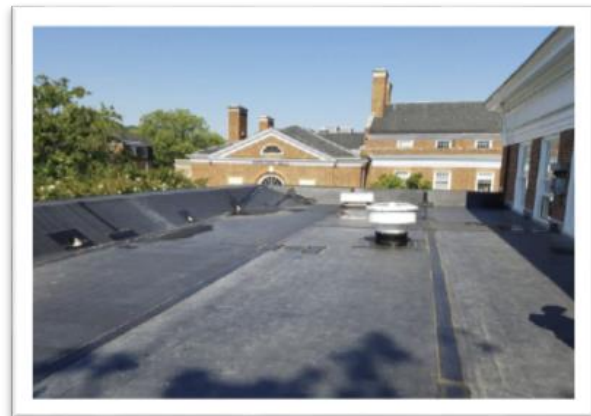
Peabody Hall Roof - After
