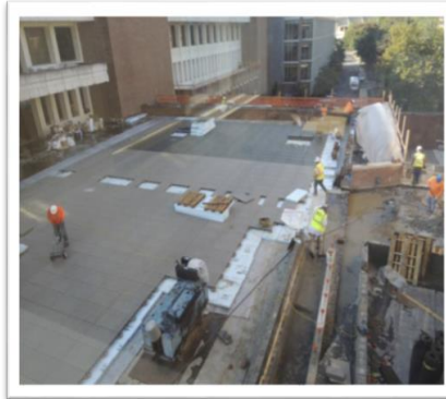
Chemistry Plaza – New water proofing and paver install
