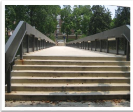
Ruffner Bridge - Before
