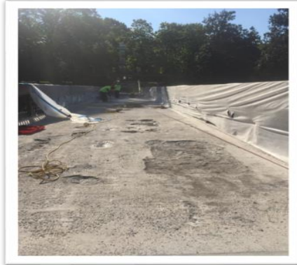
Ruffner Bridge - In progress
