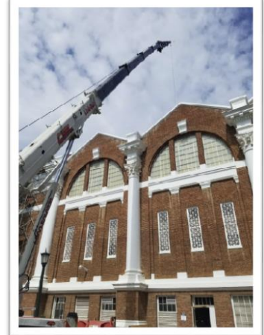
Memorial Gym Roof – In progress
