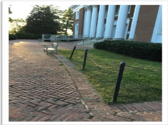
Clark Hall Plaza - Before
