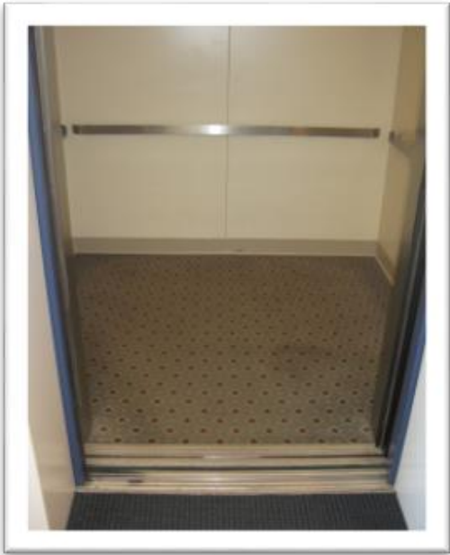
Peabody Hall – Elevator before
