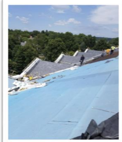
Memorial Gym Roof – In progress
