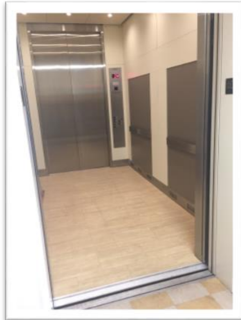
Bayly Building – Elevator Modernization Completed
