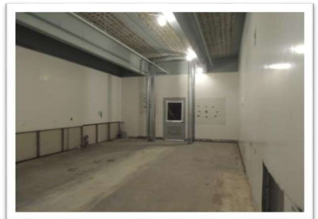
Chemistry – 2 nd floor lab framing
