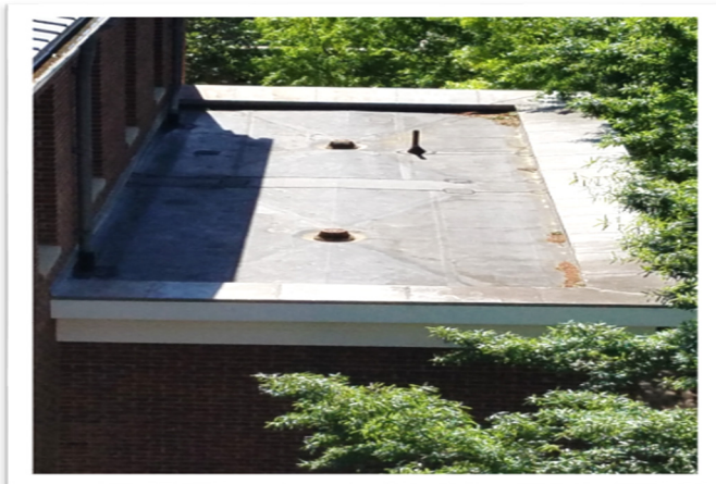
Bryan Hall – Small roof before
