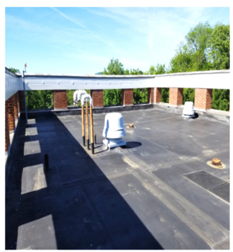
Bryan Hall – Roof before
