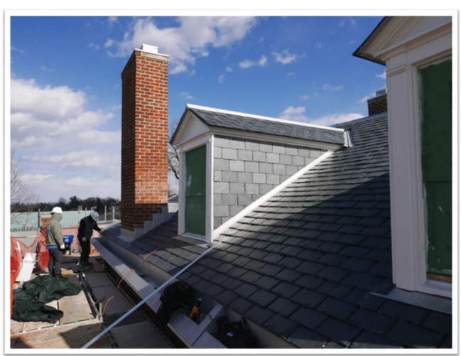
Carr's Hill President's House – Roof replacement complete
