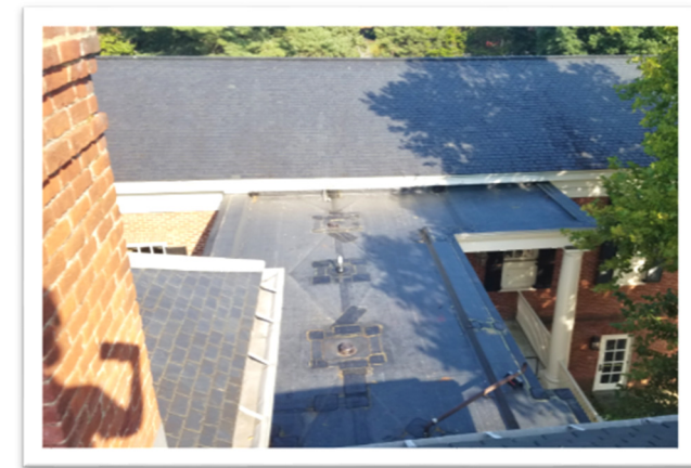
Faulkner House – Roof after
