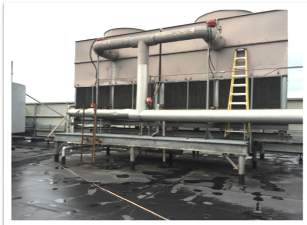
Aurbach - Cooling tower before
