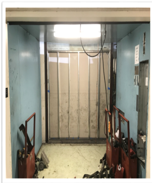
Physics Building – Elevator before
