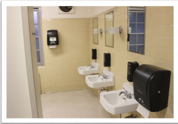
Astronomy Building – Bathrooms before
