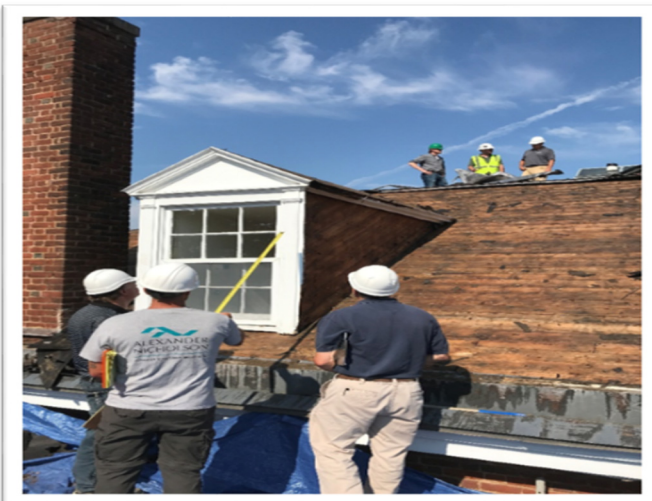
Carr's Hill President's House – Roof replacement in progress
