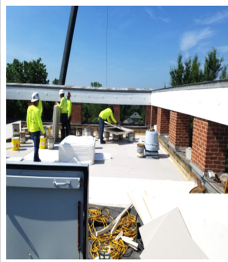
Bryan Hall – Roof in progress
