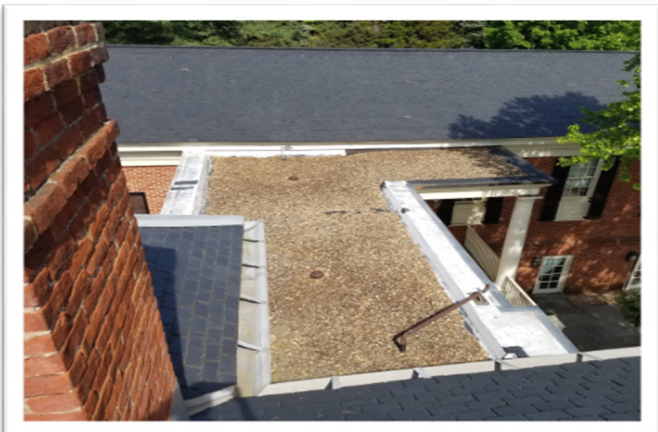
Faulkner House - Roof before
