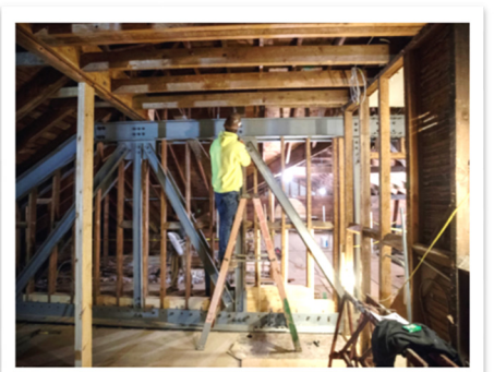
Carr's Hill President's House – Steel truss installation
