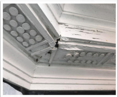
Carr's Hill President's House – Exterior trim before
