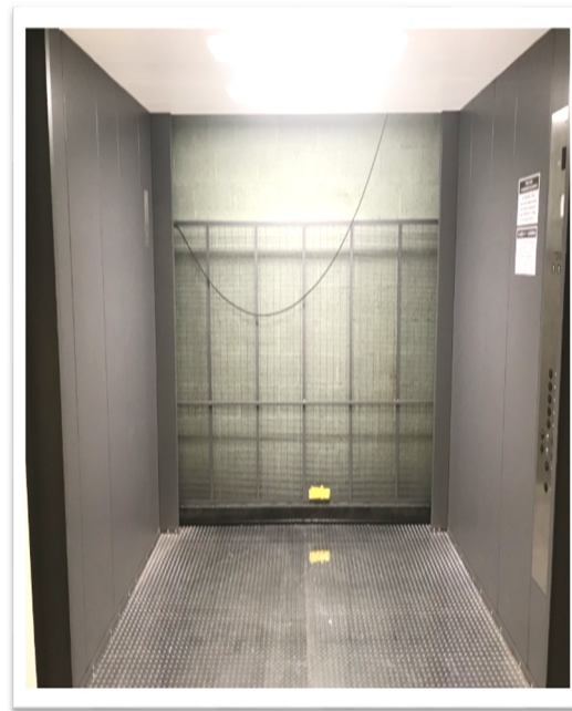
Physics Building – Elevator Modernization Completed
