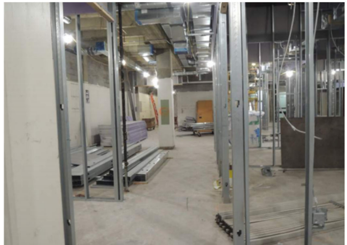
Gilmer Hall – Third floor partition framing and MEP rough-in
