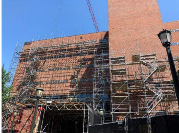
Pinn Hall – West scaffold erection
