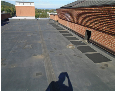
Ruffin Hall – EPDM roof before
