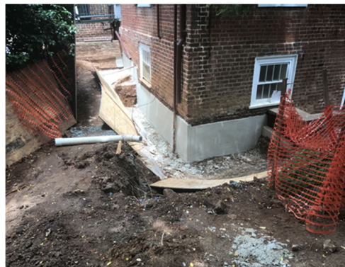
Hotel C – Drainage Improvement foundation in progress
