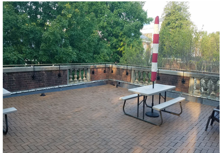
Maury Hall – Low slope roof after
