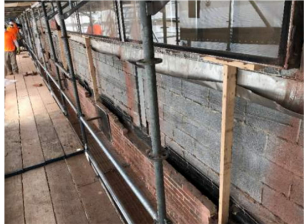
Pinn Hall – Brick veneer removal
