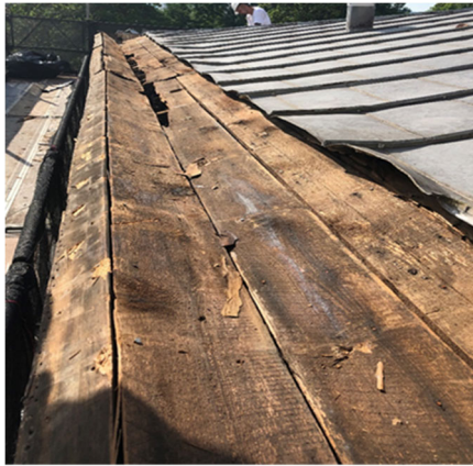
Pavilion X – Gutter & Roof repairs before
