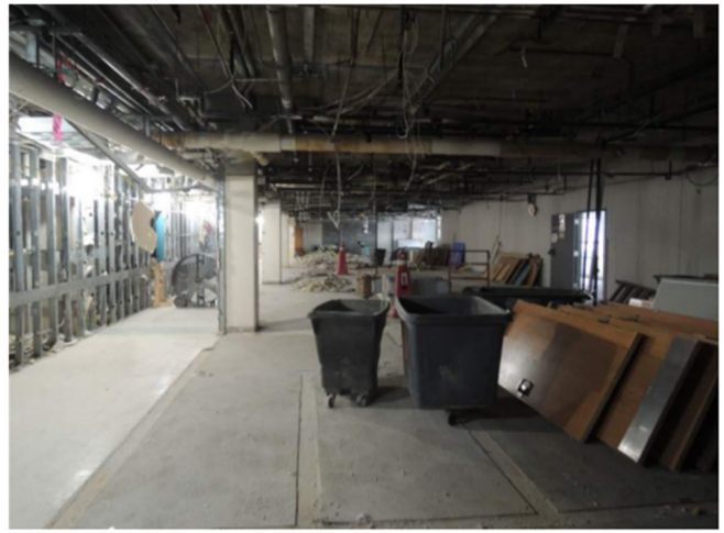
Gilmer Hall – First floor demolition in progress
