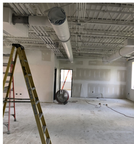
Michie Building – Renovation in progress
