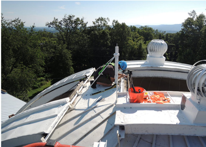
McCormick Observatory – Dome repairs
