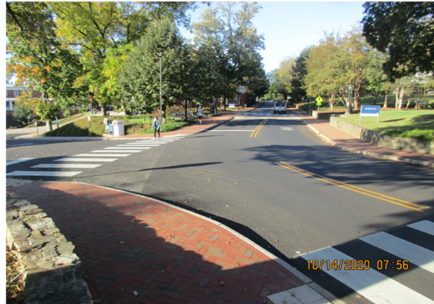
McCormick Rd – Crosswalk after
