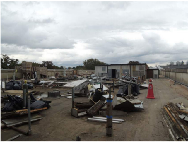
Gilmer Hall – Mechanical roof top equipment demolition
