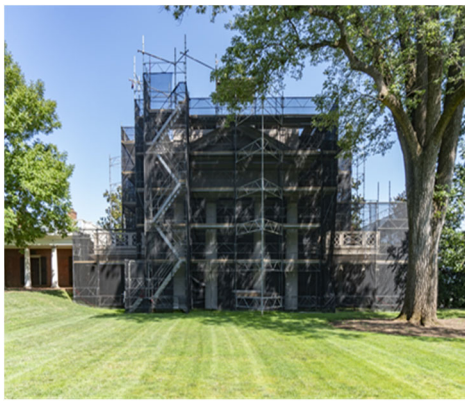
Pavilion X – Exterior repairs in progress
