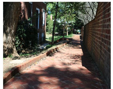
Hotel C – Drainage Improvement sidewalk after
