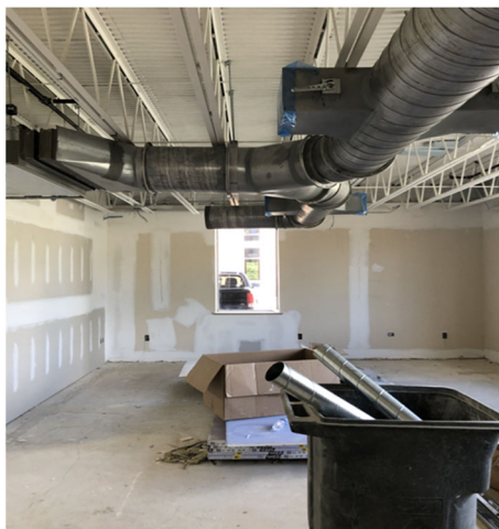
Michie Building – Renovation in progress
