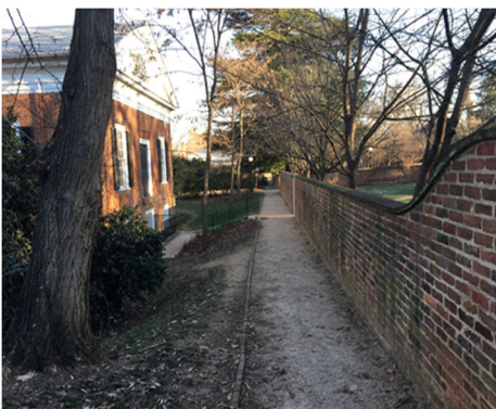
Hotel C – Drainage Improvement sidewalk before
