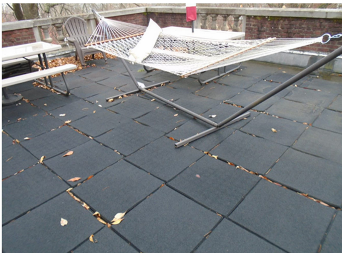
Maury Hall – Low slope roof before
