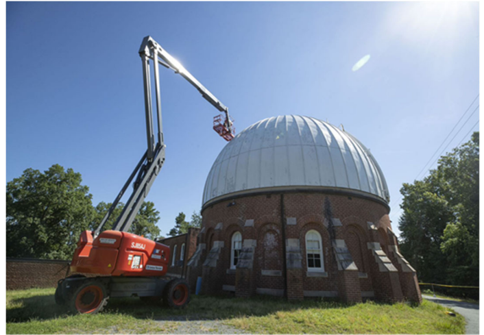
McCormick Observatory – Dome repairs
