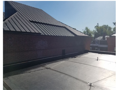
Ruffin Hall – EPDM roof after
