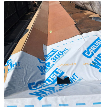
Pavilion X – Gutter & Roof repairs after
