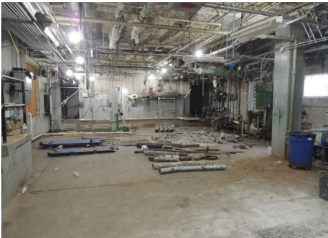
Gilmer Hall – Mechanical room demolition in progress
