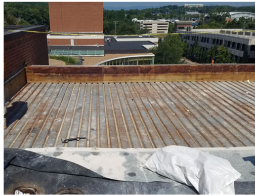
Ruffin Hall – EPDM roof replacement in progress
