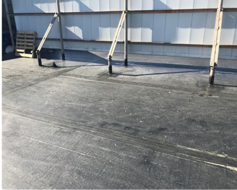
Aurbach Roof - Before
