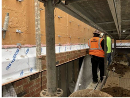
Pinn Hall – West facade brick install
