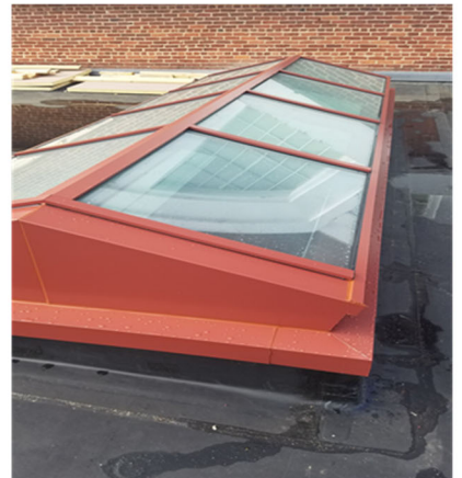
Mem Gym Skylight - After
