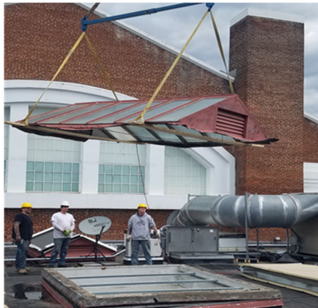
Mem Gym Skylight - Removal
