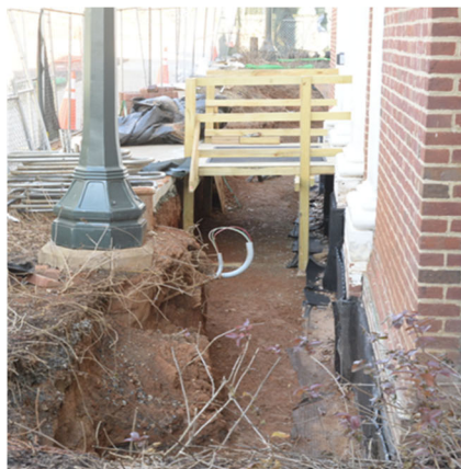
Maury Hall - Foundation waterproofing in progress (maintaining ADA access)
