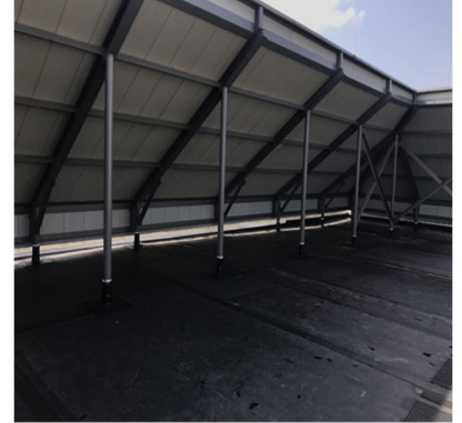
Aurbach Roof - Finished
