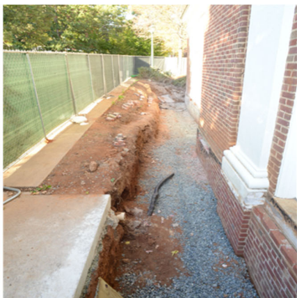
Maury Hall - Foundation waterproofing in progress
