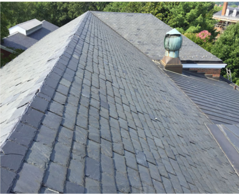
Bayly Building – Roof before
