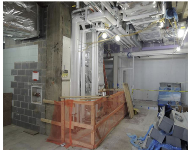
Gilmer 5 th Level – MEP installation nearing completion
