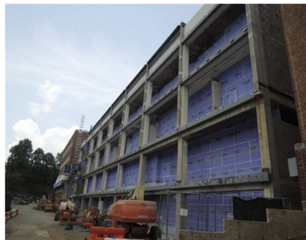
Gilmer South Facade – Precast and curtainwall infrastructure in place
