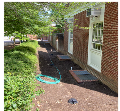
Maury Hall - Foundation waterproofing completed
