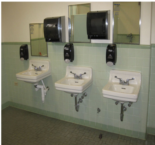
Zehmer Hall – First floor bathrooms – before
