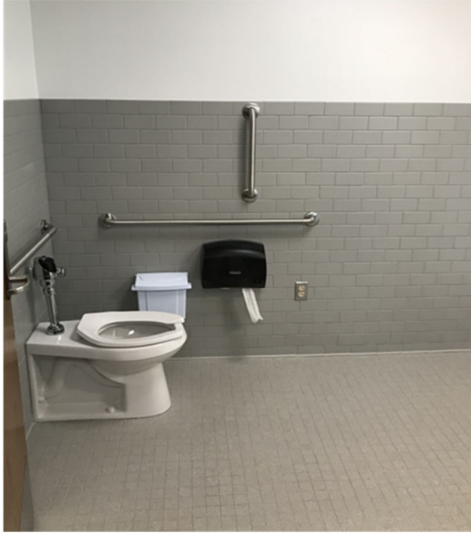
Fiske Kimball – New first floor ADA Bathroom
