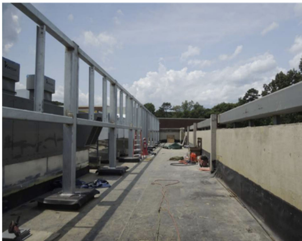
Gilmer Central Roof – New structure for screen wall
