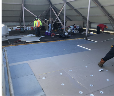
Aurbach Roof - In-progress
