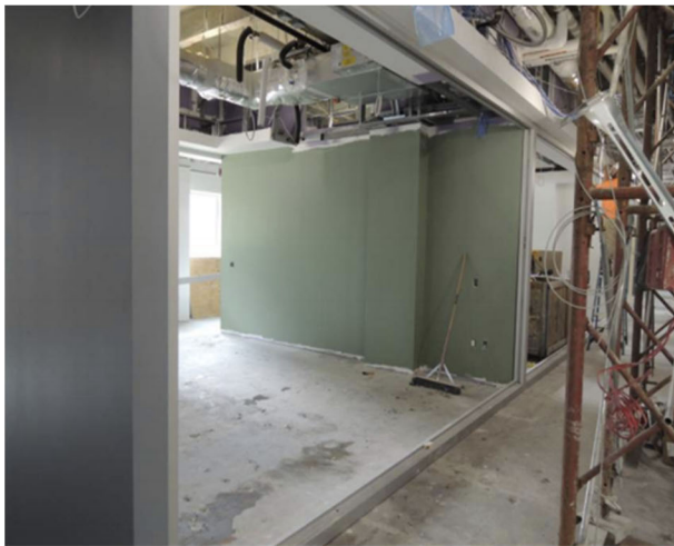
Gilmer 5 th Level – Interior storefront in-progress
