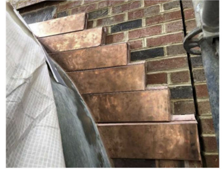
Pinn Hall – North façade step flashing
