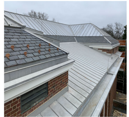
Bayly Building – Roof completed
