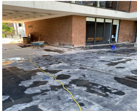
Campbell Hall Plaza - In progress
