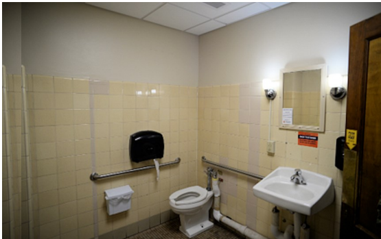
John Warner Hall - 1st Floor restroom before
