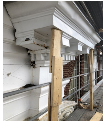
Mem Gym - Cornice before
