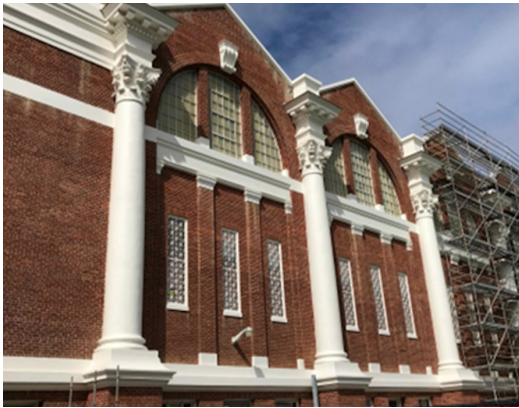
Mem Gym - Exterior Renewal in progress
