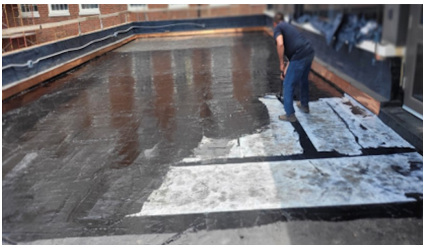
Clemons Library Plaza - In progress
