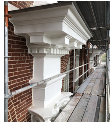
Mem Gym - Cornice after
