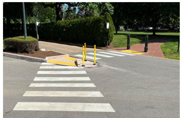
Hospital Drive - After
