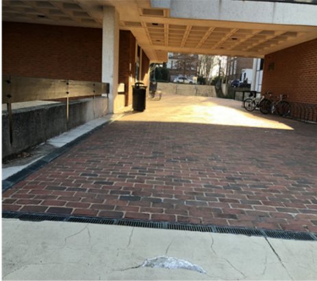
Campbell Hall Plaza Phase II – Before
