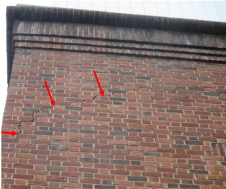
North Chiller Plant – West exterior wall - Before
