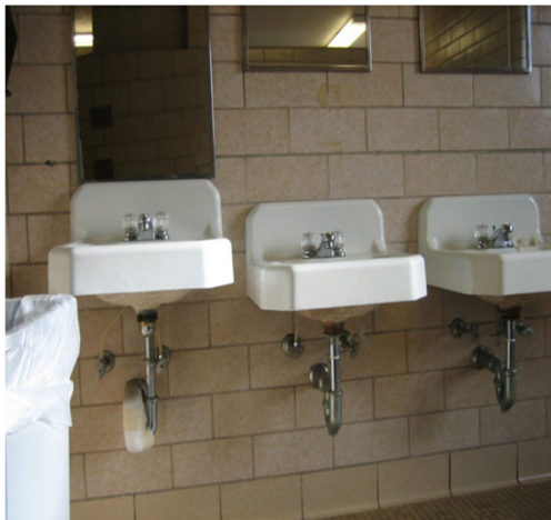
Kerchof Hall – Bathrooms - Before
