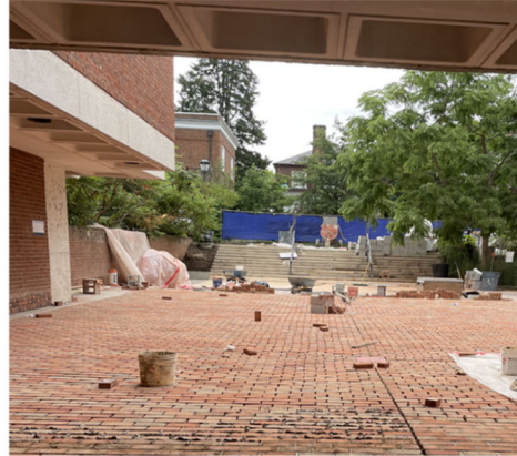
Campbell Hall Plaza Phase II – In-Progress
