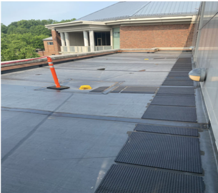
Chemistry Addition – New Roof
