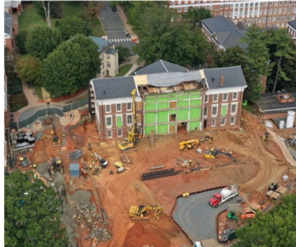
Cobb Hall – Exterior – In-Progress
