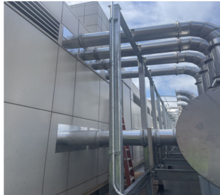
Chemistry Addition – New exhaust stacks
