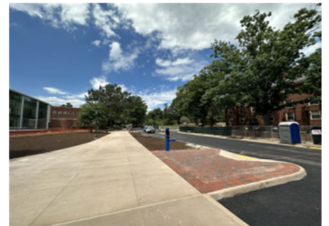
McCormick Rd – Sidewalk condition - After
