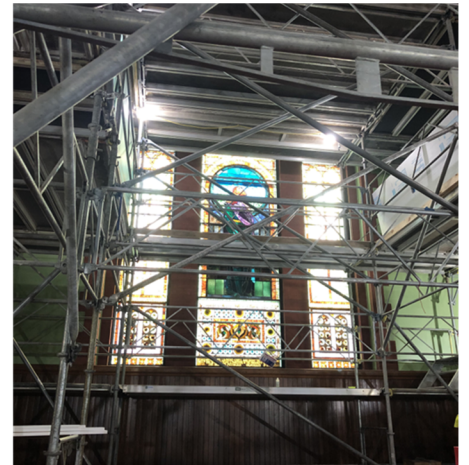
University Chapel – Interior renovation – In-Progress
