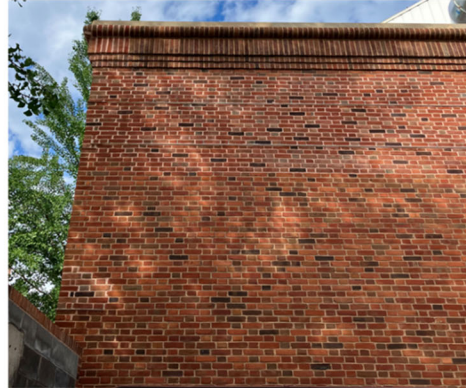
North Chiller Plant – West exterior wall - After
