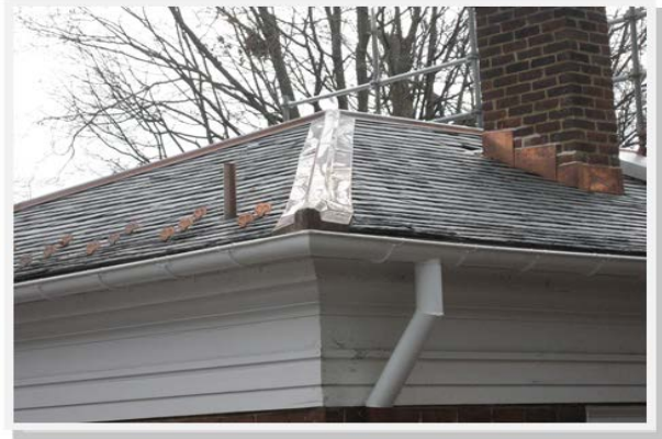
East Range – Roof after
