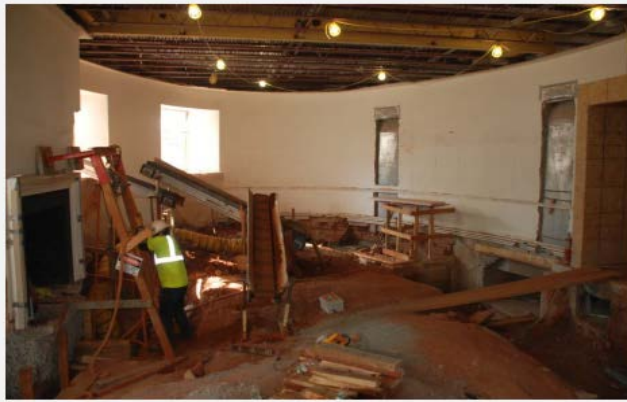
Rotunda – East oval room selective demolition
