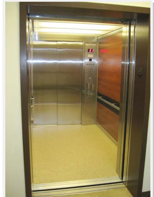
Thornton Hall E-wing - Modernization completed
