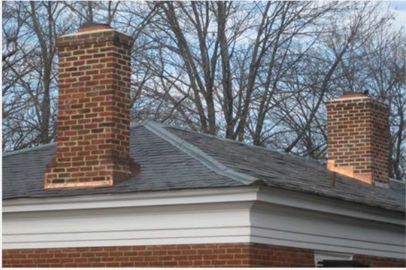
East Range – Roof before
