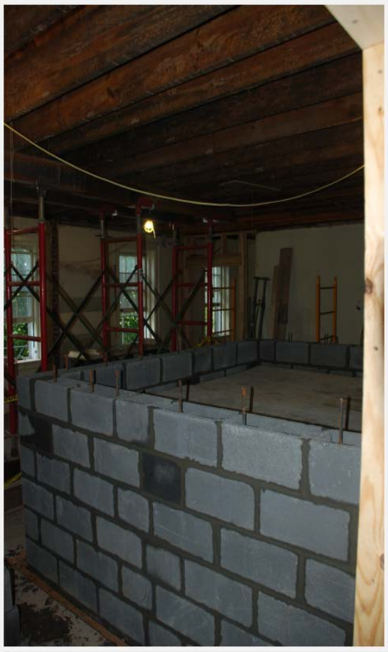
Rugby – Elevator shaft being constructed
