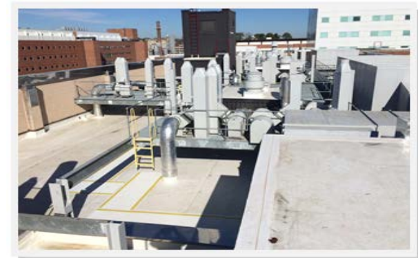
MR-4 – Roof after
