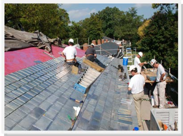
Hotel D – Roof in-progress
