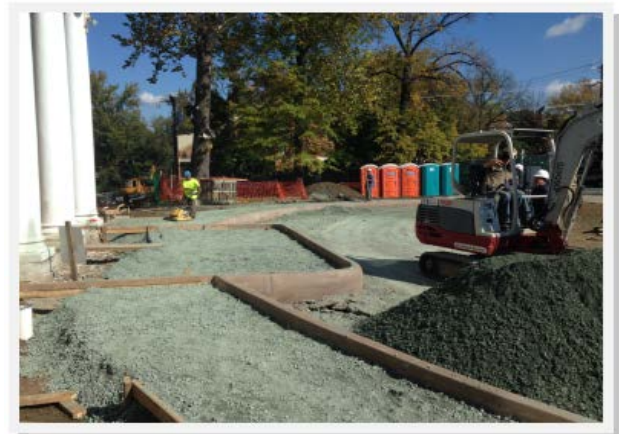
Rugby – Curb installation
