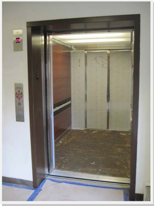
Thornton Hall E-wing - Modernization in progress
