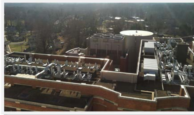
MR-4 – Roof before
