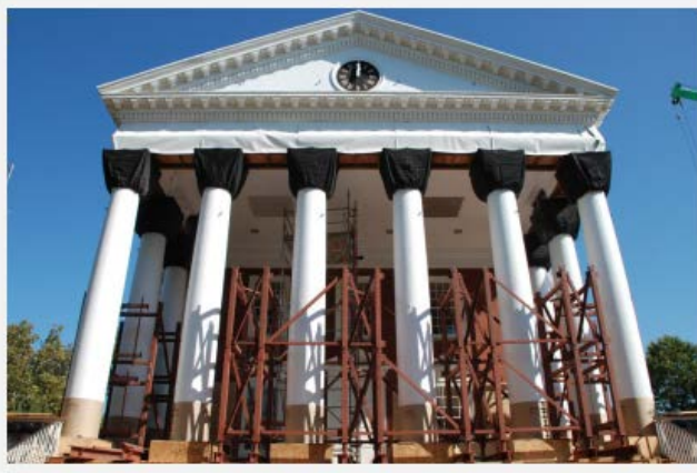
Rotunda – Steel shoring for capital replacement
