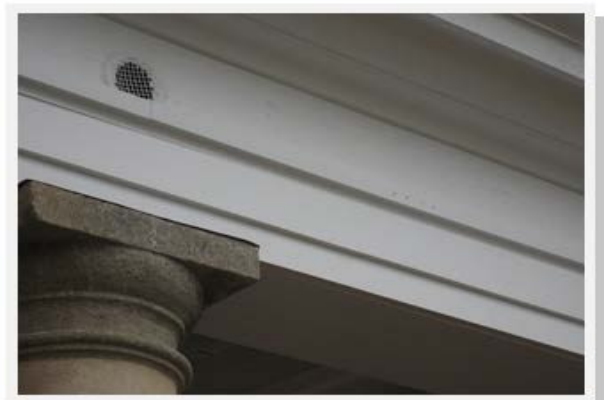
East Lawn – Colonnade support beam partial repair
