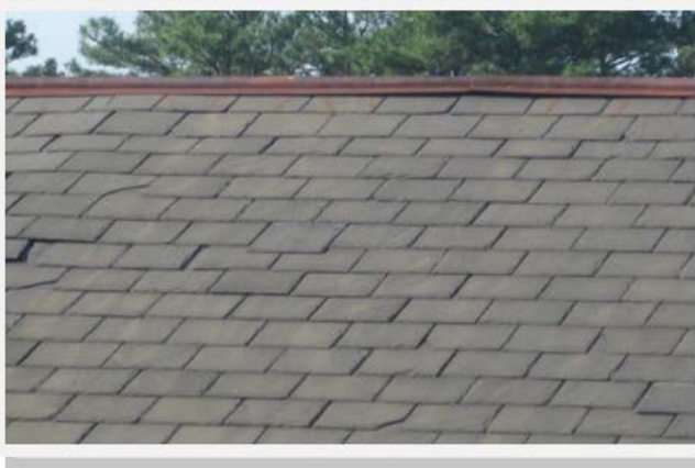
McIntire Wing – Roof before
