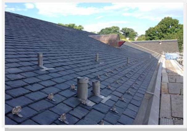
McIntire Wing – Roof after
