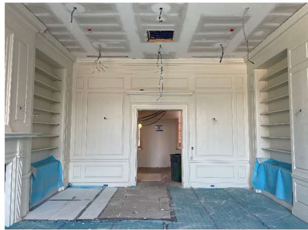
Garnett Room restored, new ceiling install, freshly painted.
