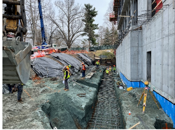
Start work on north terrace.
