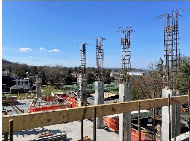
Rebar ready for Level 5 column forms
