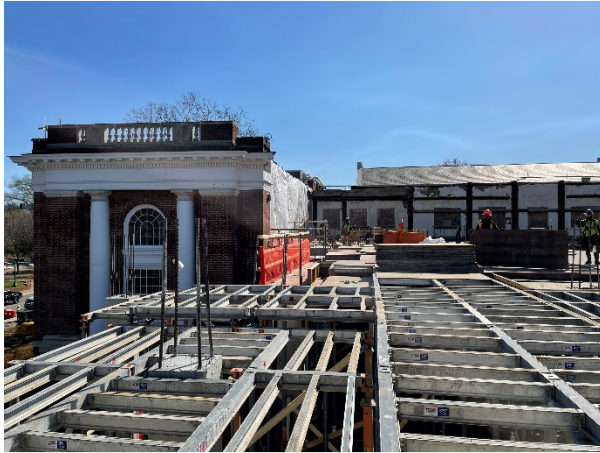
Decking formwork for Level 5 floor slab
