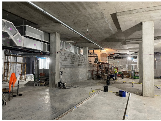
New Addition, interior walls, overhead MEP, and Rails for Compact Shelving
