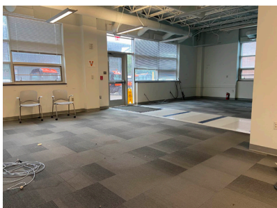
The start of the Skipwith Hall lower level renovation, June 2023. Photo provided by Emily Douglas.
