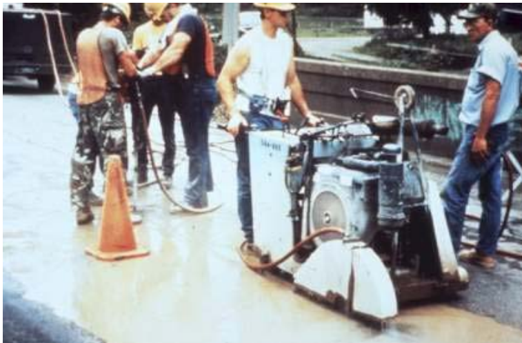
Using water to cut concrete and bricks
