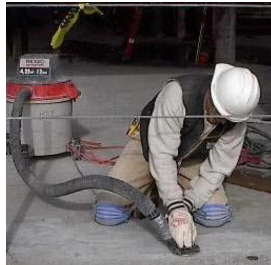
Concrete sander with exhaust ventilation
