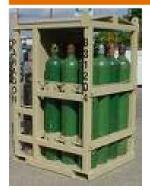
Storage: Cylinders must be secured to prevent tipping.
