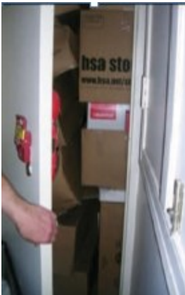
Emergency exit routes must be clear of all obstructions
