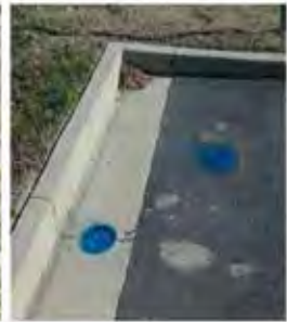
Valve box cover marking
