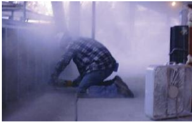
Using a grinder in poorly controlled conditions. (Photo courtesy of the University of Washington.)
